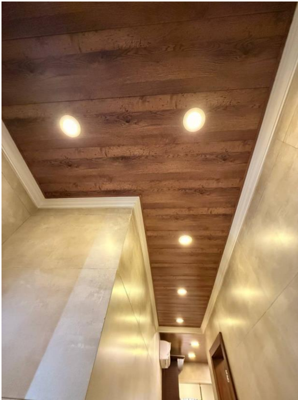
Figure 9 - Kitchen Corridor Ceiling
