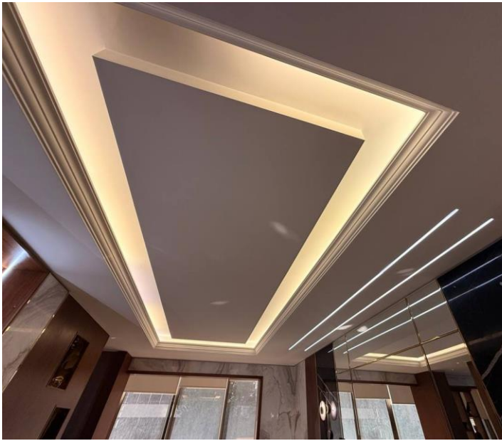
Figure 13 - Dining Room Ceiling
