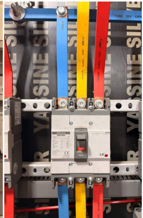
Figure 6 - Hashem three-phase MCCB, handle marked 150 A. Fun Fact: NOTICE 3-PHASE COLORS OF INDIA's National Code, as per in the slides.
